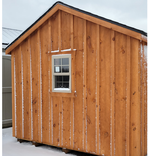
1 X 12 KILN-DRIED WHITE PINE BOARD & BATTEN SIDING WITH KNOTS
